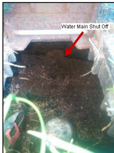
Water Shutoff and Meter (Located next to Mailbox)
