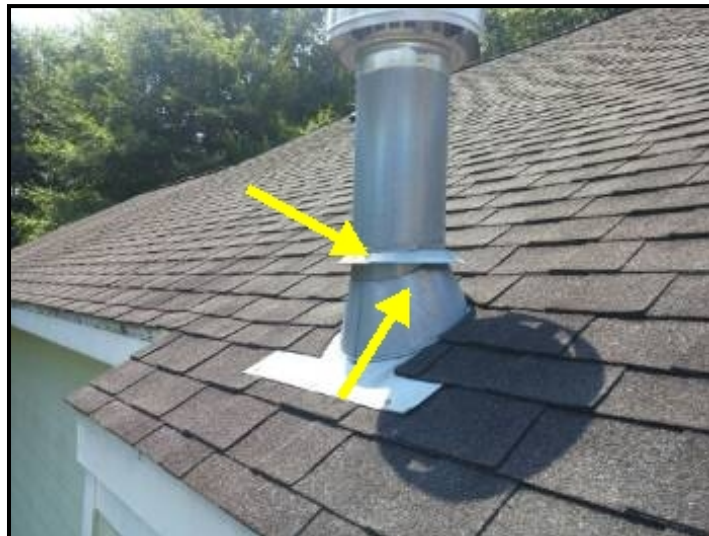
Caulking is needed, Water is coming through
