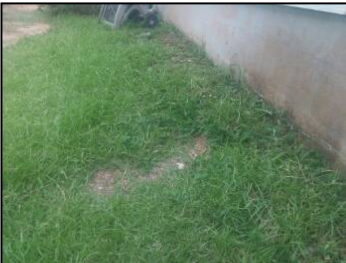
Storm water not draining properly from foundation.
