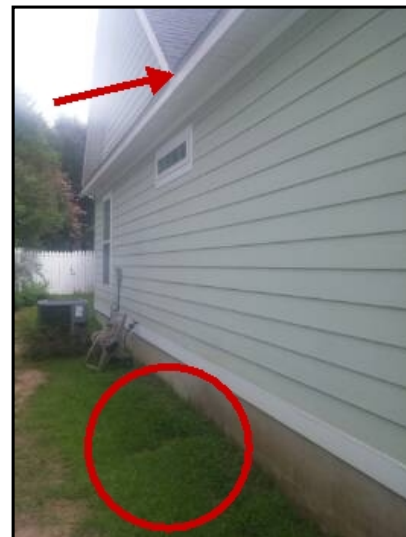
Grading is worse at valleys.
