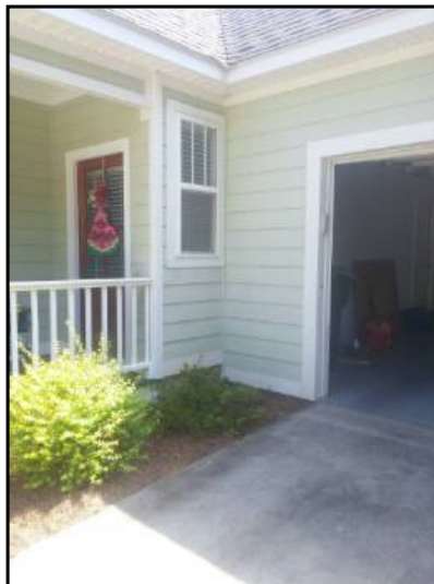
Water runoff is too close to foundation. Gutters are recommended
