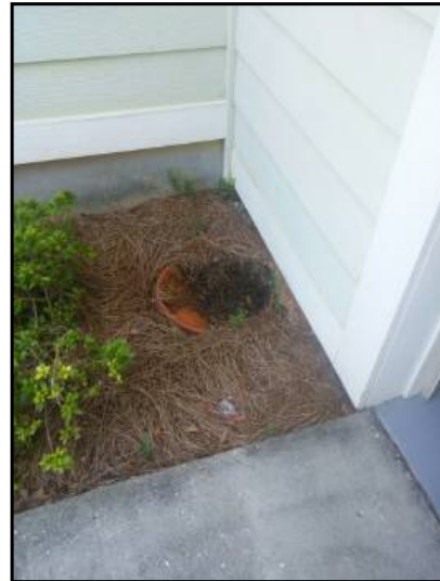
Water runoff is too close to foundation. Gutters are recommended
