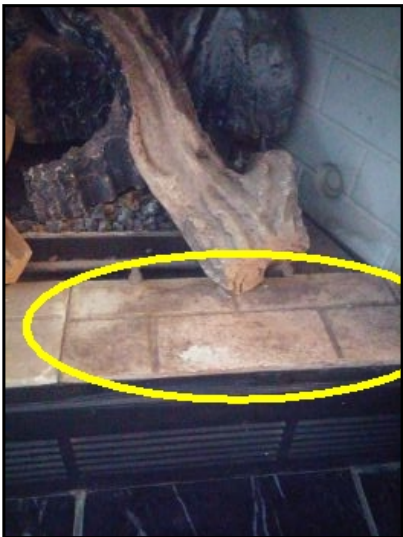
Leak from uncaulked flue
